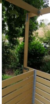
Recycling bin shelter
